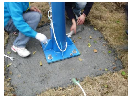
Screw down two nuts on each bolt.
