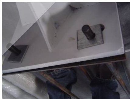
Lifting the pole with crane and put it on the underground work.
